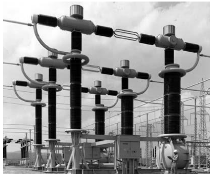
Gambar 6.10. Air Circuit Breaker
